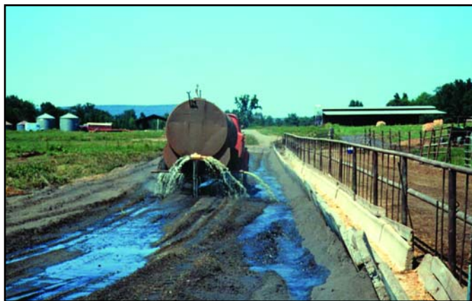
Watering of mixture of fly ash and soil during placement and compaction.
