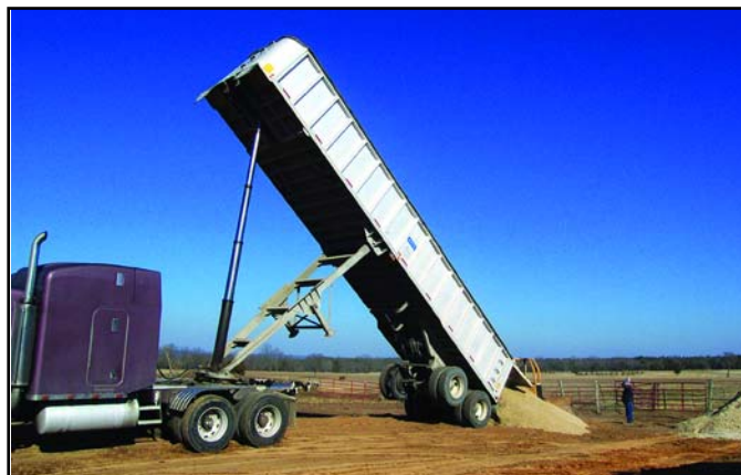
Blend of bottom ash and fly ash being delivered to the heavy use area. The existing top layer of manure and mud has already been removed and land applied.
